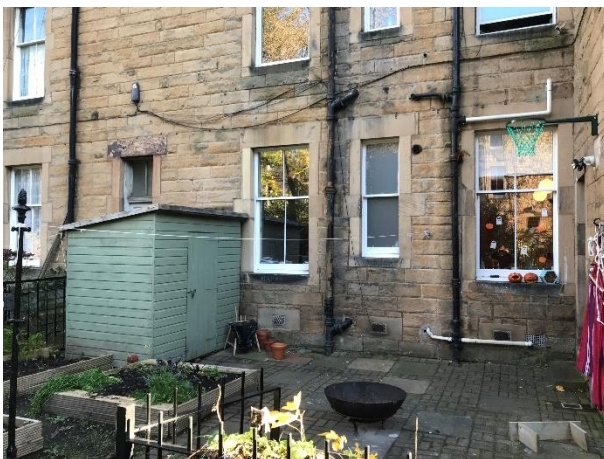
Existing private back garden and rear elevation
